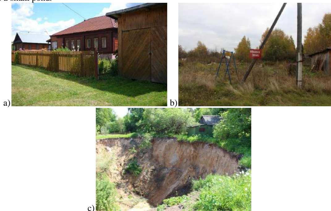
Figure 1. Sinkhole in village Chud: a – The place of sinkhole in 2013, b – The place of sinkhole in 2014, c – State of sinkhole in the summer of 2014.
